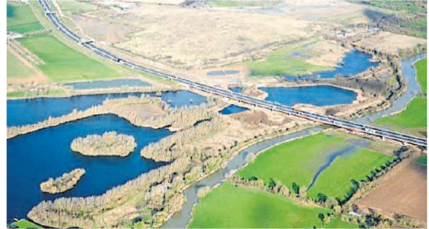
Vehicles using the 750-metre long River Great Ouse viaduct on the new A14
