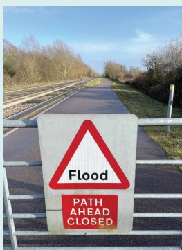
Busway path section flooded
